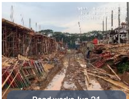
Road works Jun 21
